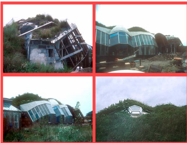
Large earth shelter house from recycled materials under construction.
